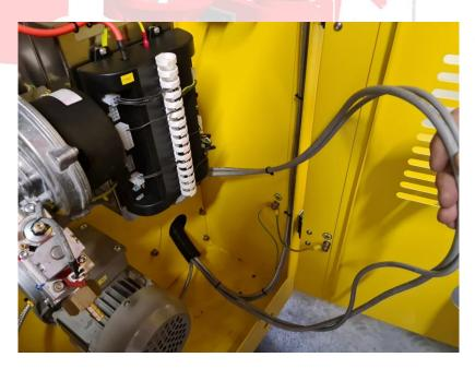
Cut the zip ties and unwind the cable
